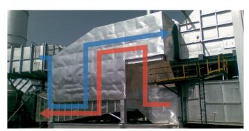
New arrangement with REKULUVO, no unexpected shutdowns, zero maintenance, achieved energy saving 134,000 MMBTU/a (39,260 MW/a)\*\*
