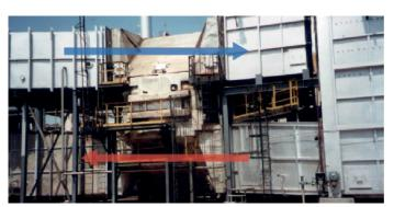
Prior arrangement with rotary regenerative type, several unexpected shutdowns and 15% leakage
