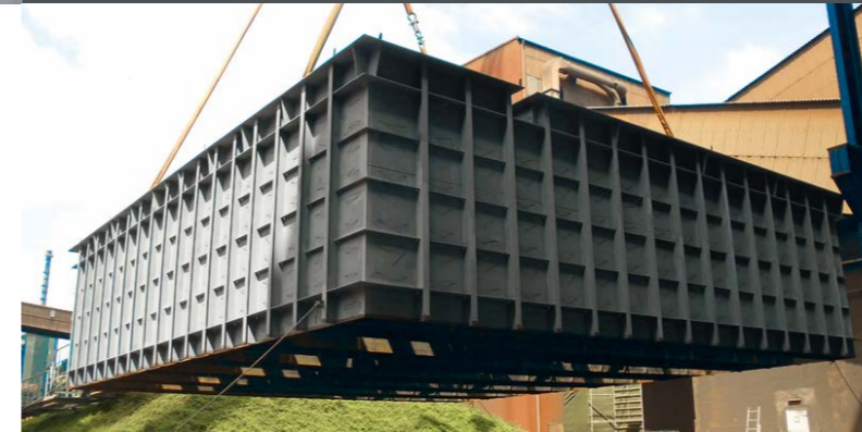
Transport and erection demand maximum commitment and expertise
