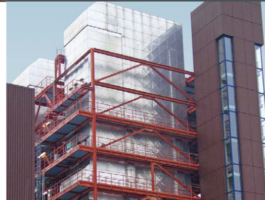
Proven use in waste incineration plants
